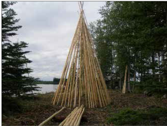
Spruce poles drying to construct a fish wheel at a fish camp on the Tanana River, Yukon Area. © ADF&G. Photo by Bonnie Borba.
