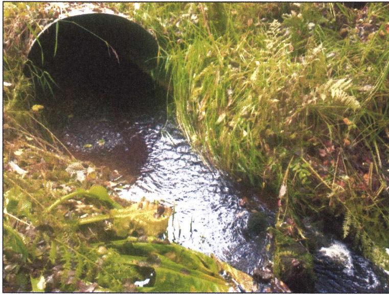
Figure 1.—Culvert outlet at waypoint 2501.
