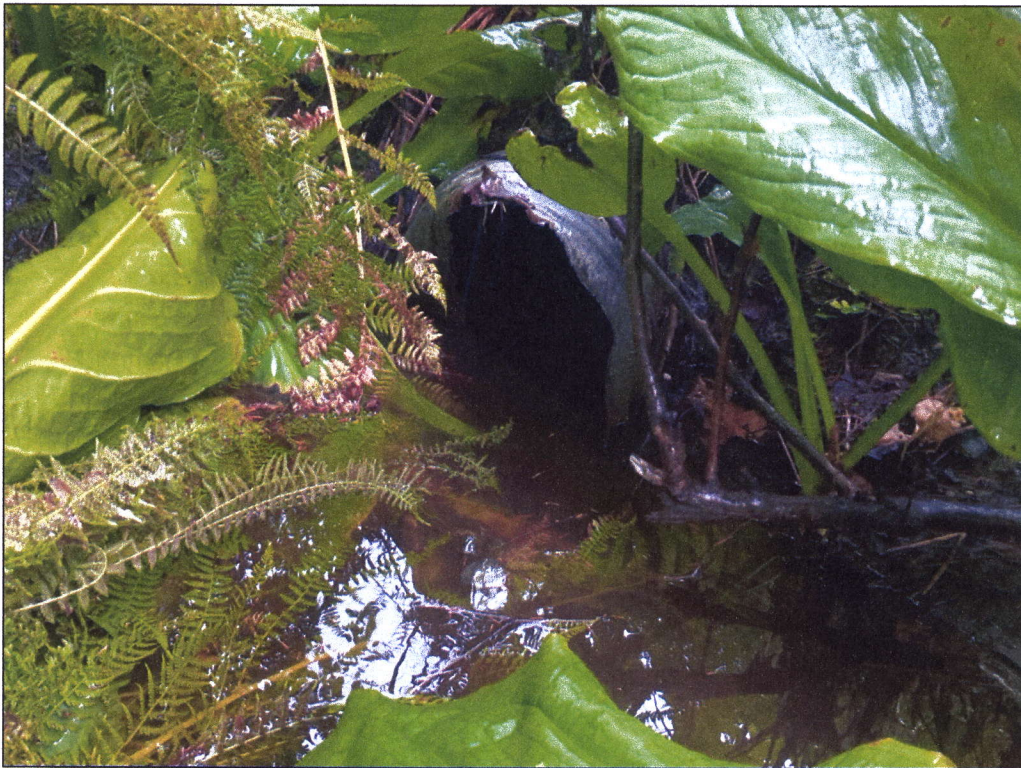
Figure 2.—Partially crushed culvert outlet at waypoint 1653.
