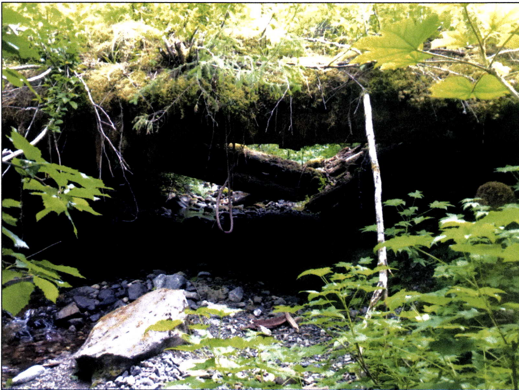
Figure 3.—Partially collapsed log-stringer bridge at waypoint 936.
