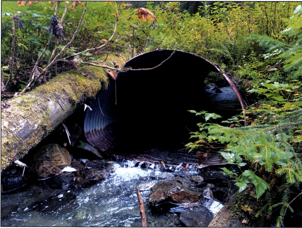
Figure 2.—Culvert outlet at waypoint 1785.
