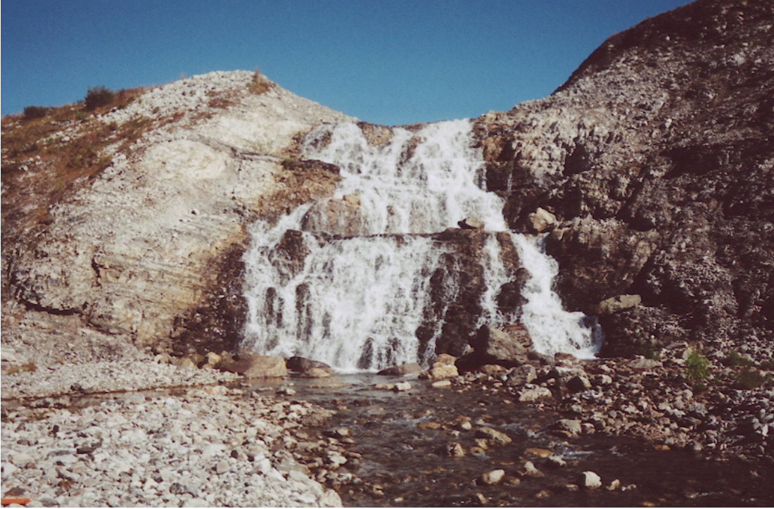
Figure 22. Spillway at the end of the bypass channel carries water around Bons Pond dam.
