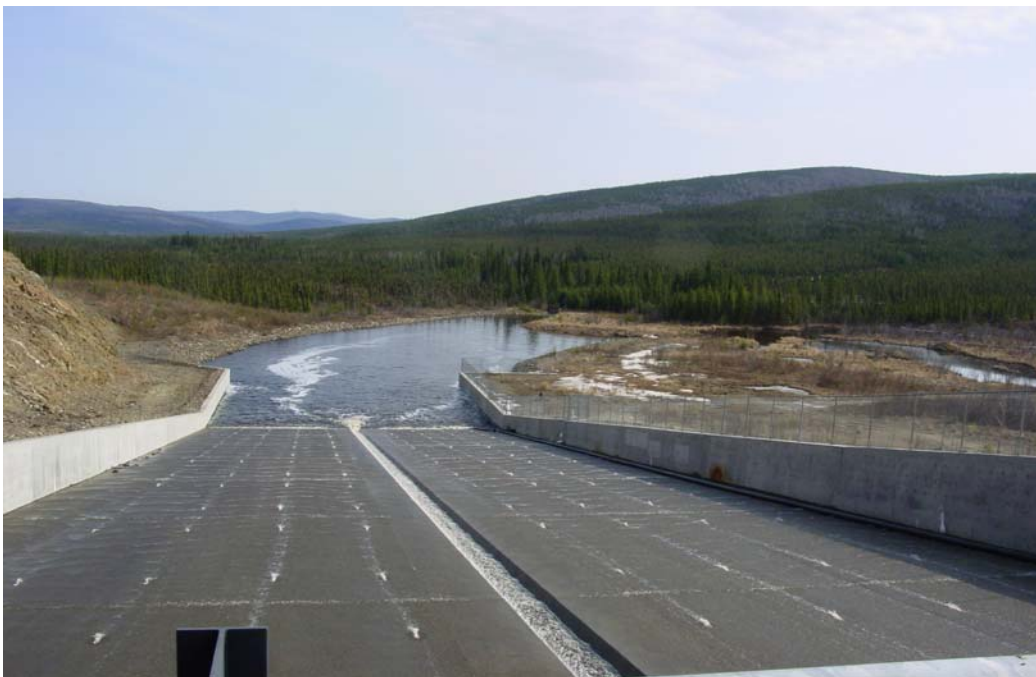
Figure 5. Spillway, looking downstream, in Ft. Knox freshwater dam (May 2009).
