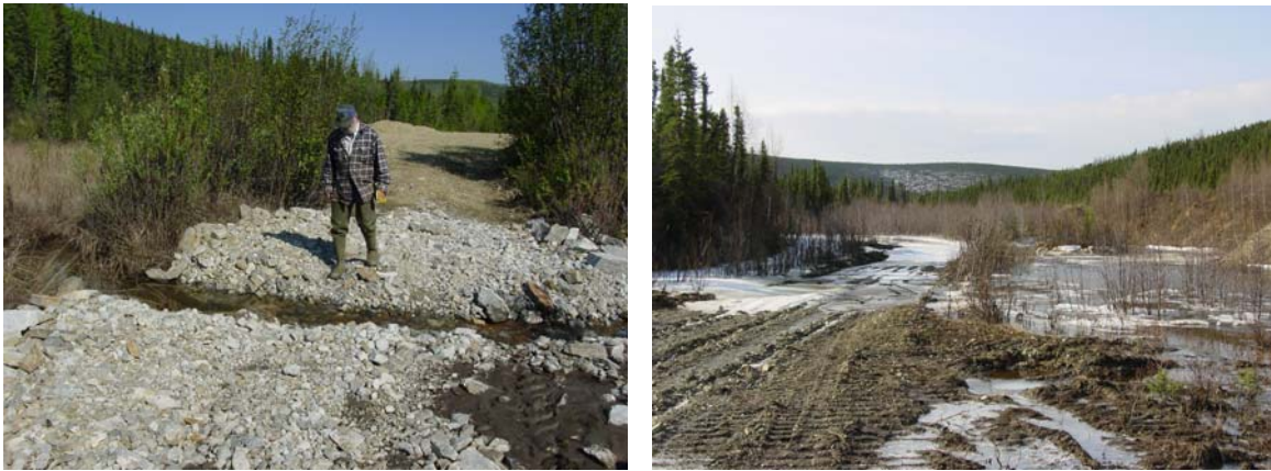
Figure 2. Reconstructed road crossings (photo on left, no aufeis) and (photo on right, extensive aufeis) June 8, 2009.
