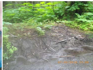
Figure 36: Bank and riparian disturbance on Little McGinnis Creek Tributary.
