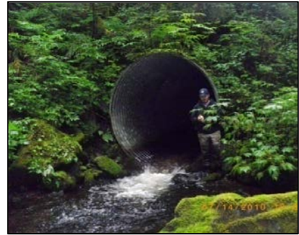
Figure 7: Field staff at culvert on Bessie creek.
