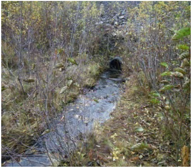
Figure 9.—Culvert draining WT-6.
