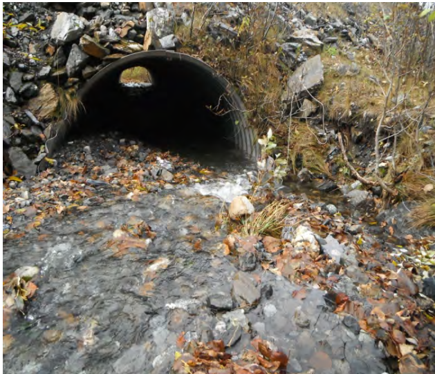
Figure 32.—Culvert CV-11 inlet.
