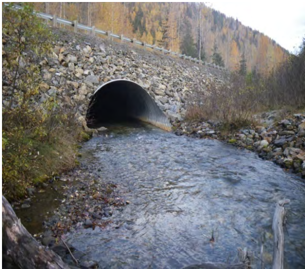
Figure 28.–Culvert CV-9 inlet.
