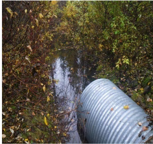
Figure 27.–Culvert CV-8 outlet.
