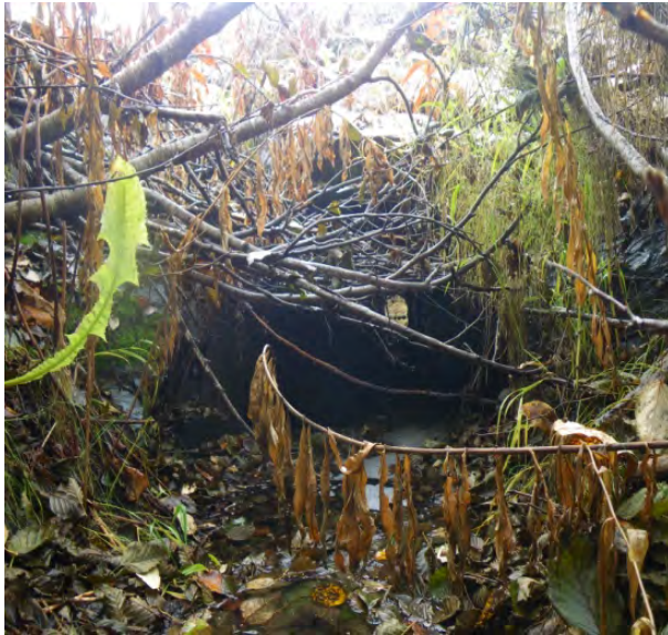
Figure 30.–Culvert CV-10 inlet.
