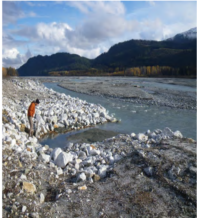
Figure 22.—Fill material placed near CV-6.
