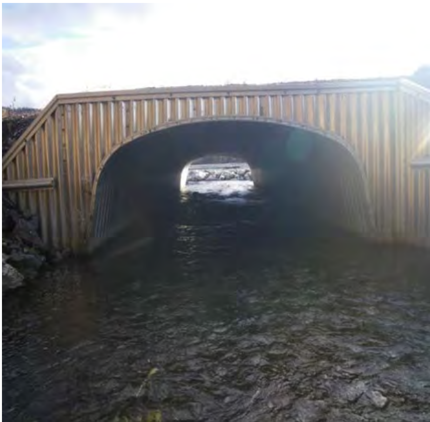
Figure 23.—Inlet to culvert CV-7.
