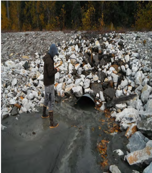
Figure 21—Outlet of culvert CV-16.
