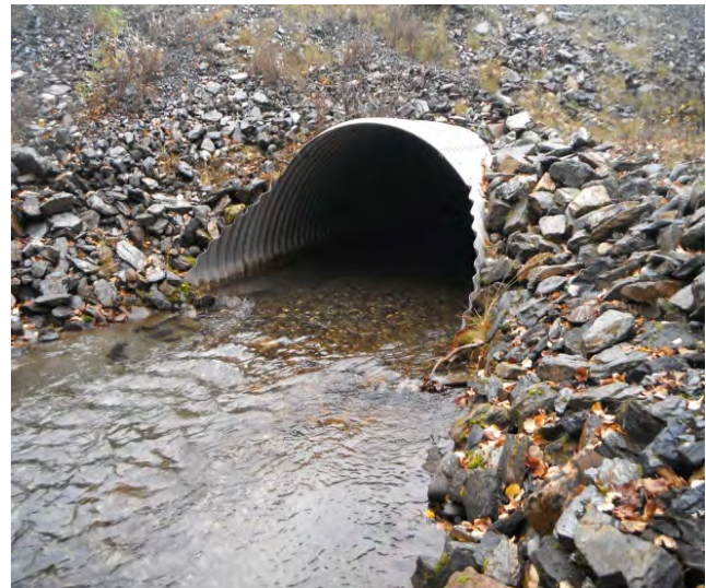
Figure 29.–Culvert CV-9 outlet.
