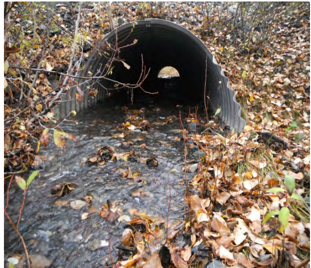
Figure 33.—Culvert CV-11 outlet.
