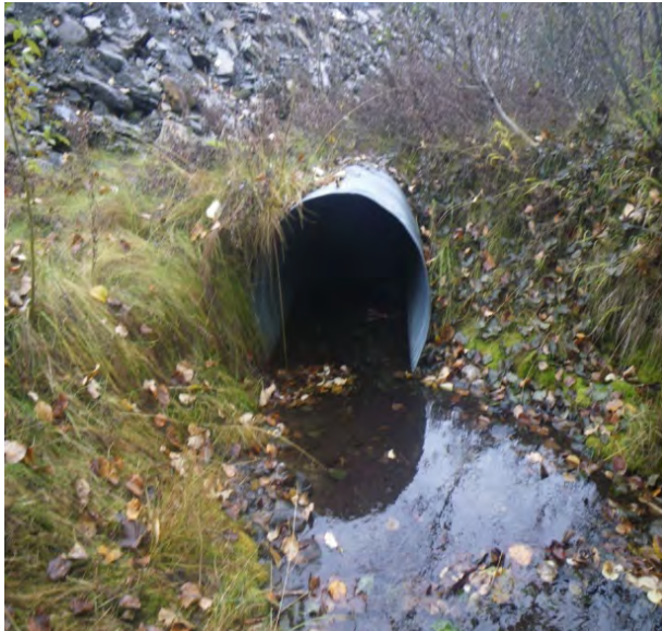
Figure 26.–Culvert CV-8 inlet.
