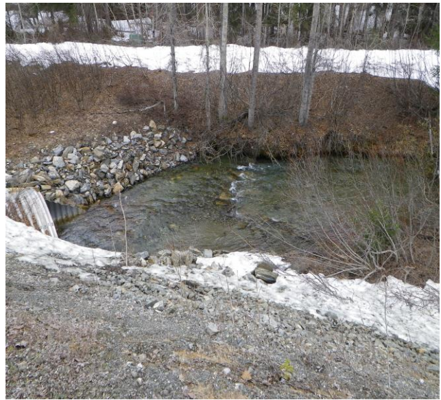
Figure 7.–Culvert CV-9 outlet 5/10/12.
