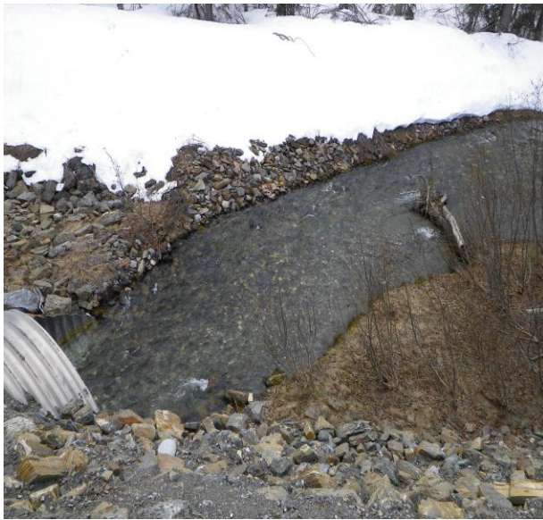
Figure 6.–Culvert CV-9 inlet 5/10/12.
