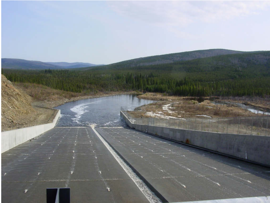
Figure 3. Spillway, looking downstream, at the Fort Knox freshwater dam in spring 2009.
