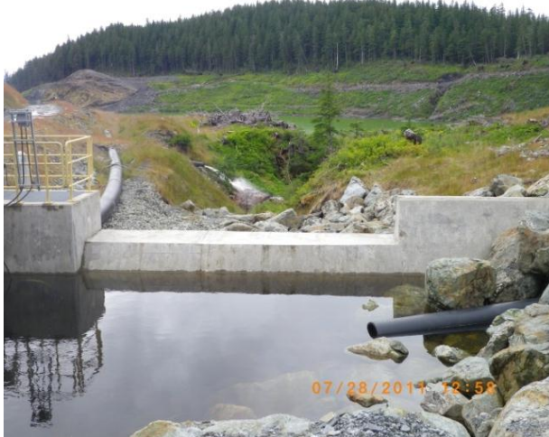
Figure 19.—Diversion dam, pipeline, and TTF.
