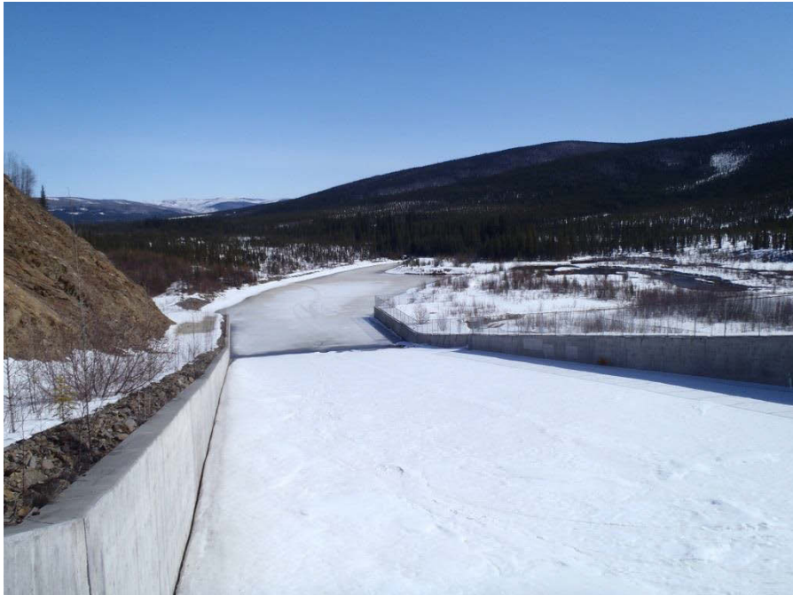
Figure 6. Spillway, looking downstream, at the Fort Knox freshwater dam in spring 2013.
