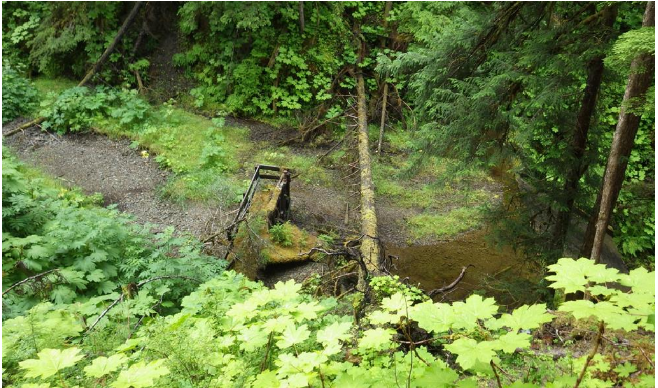
Figure 2.—Looking down at Shotter Creek immediately upstream of the dam.
