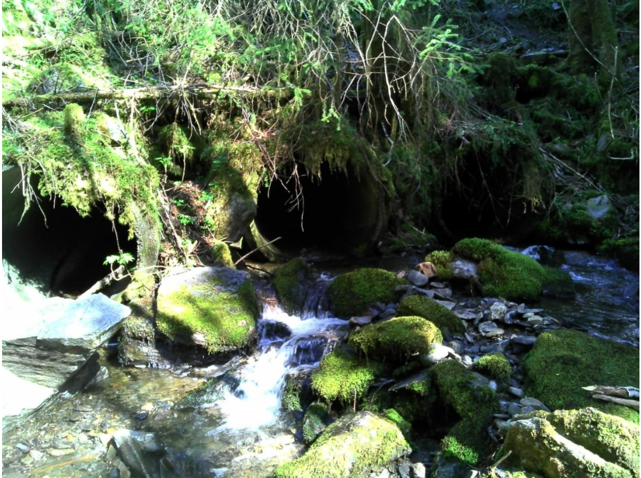
Figure 1.—Battery of 3 concrete culverts on 101-47-10150-2035.
