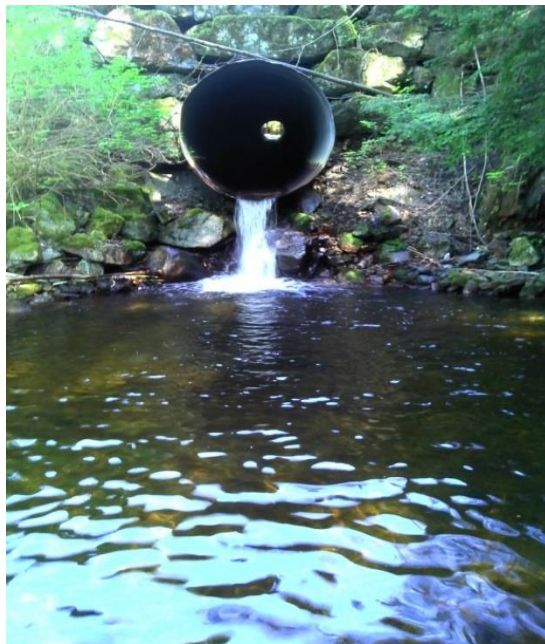
Figure 1.–Hoadley Creek barrier culvert.
