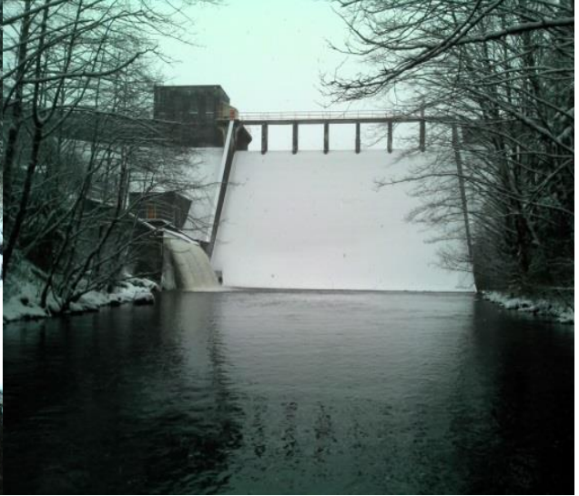
Figure 2.—Dam on Ward Creek.
