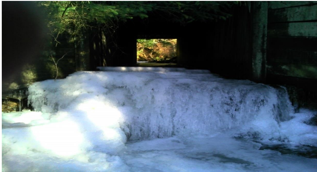
Figure 1.–101-47-10300 culvert barrier in the winter.
