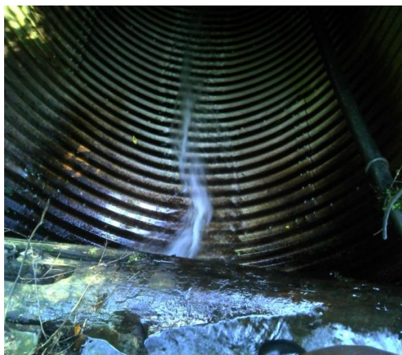
Figure 1.–Perched stream with intake line.
