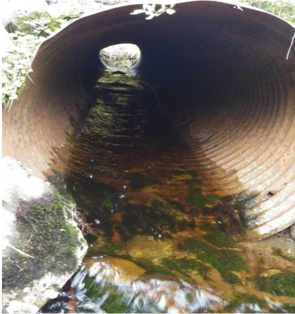
Figure 1.—Culvert outlet.
