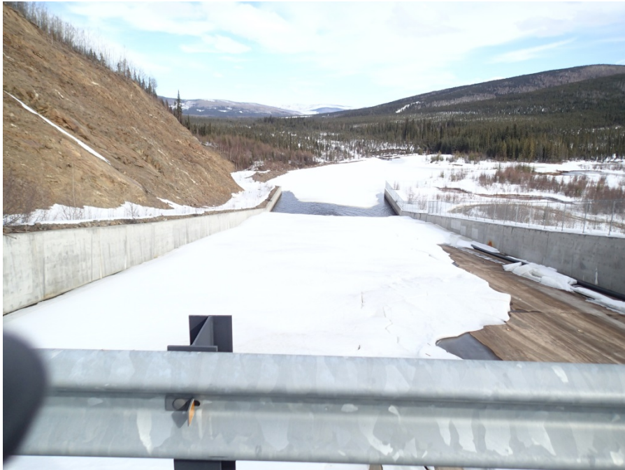
Figure 6. Stilling basin located immediately below the spillway, looking east (April 2015).
