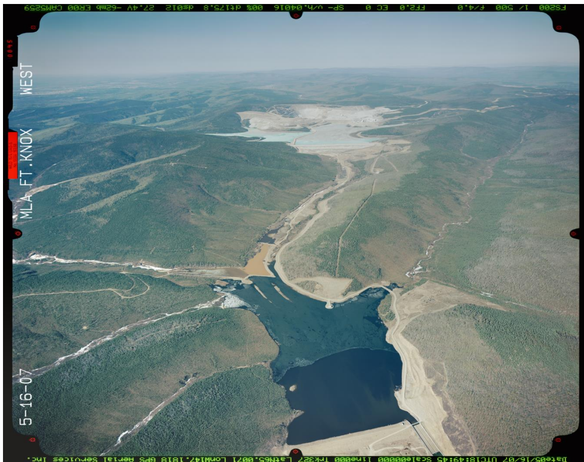
Figure 1. Aerial photograph of the Fort Knox Gold Mine WSR, tailings facility and pit – water supply reservoir in lower part of photo and the tailings dam and impoundment in the upper Fish Creek valley, photograph provided by FGMI.
