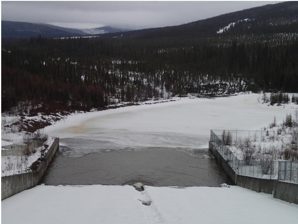
Figure 14. Stilling basin on March 29, 2016 (photo by Parker Bradley).
