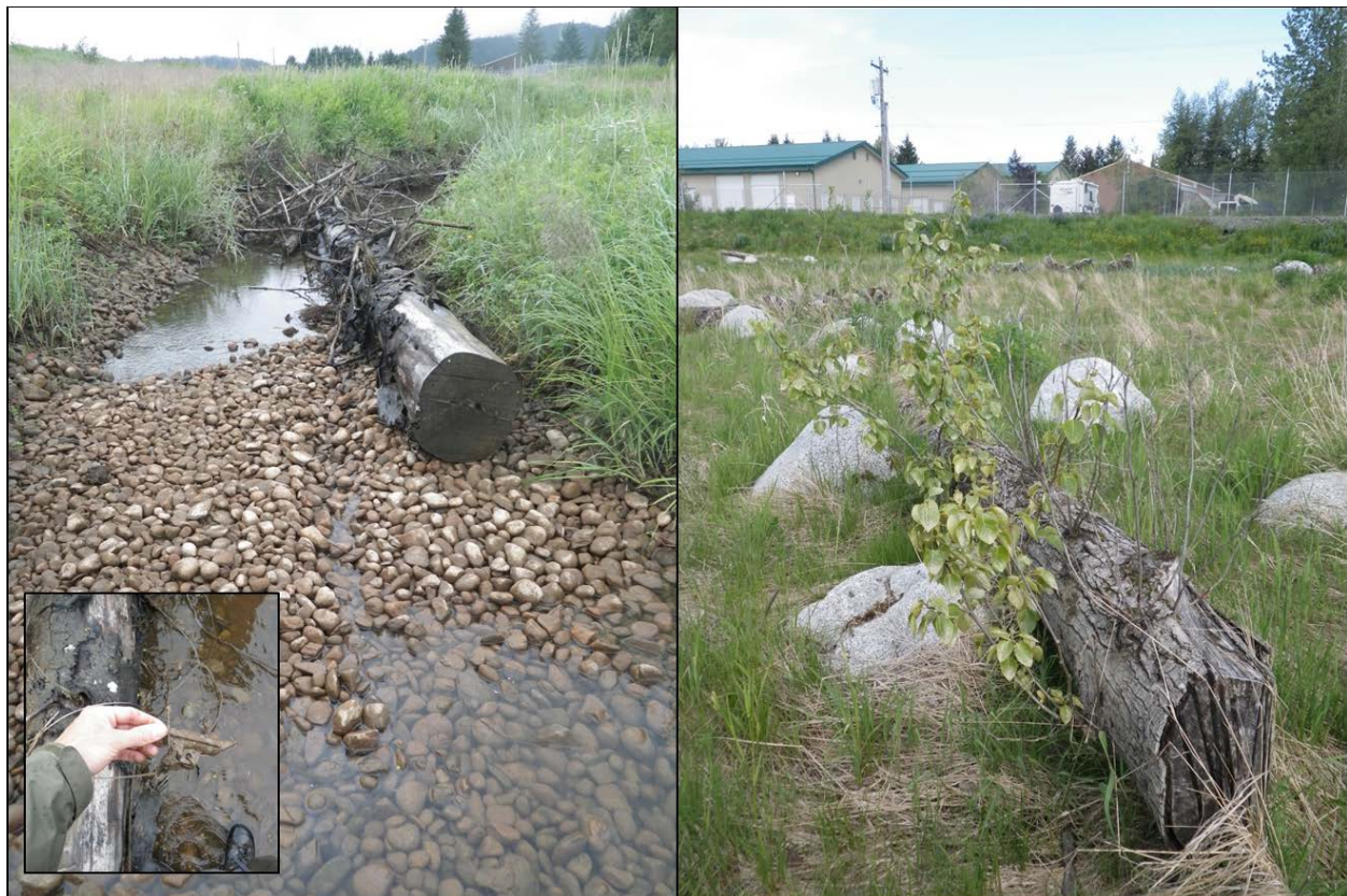
Figure 23.—Spruce tree anchor (inset) failure (left) and floodplain cottonwood (right).
