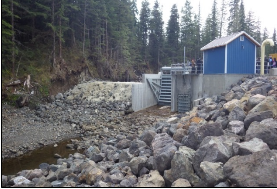
Figure 2.—Spillway, intake chamber, and sluice and radial gates.
