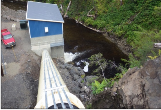
Figure 3.—Looking down the penstock at the powerhouse and bypass reach.
