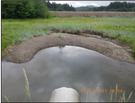
Figure 16.—Inlet of Shotter Creek culvert pre-construction, June 2011.
