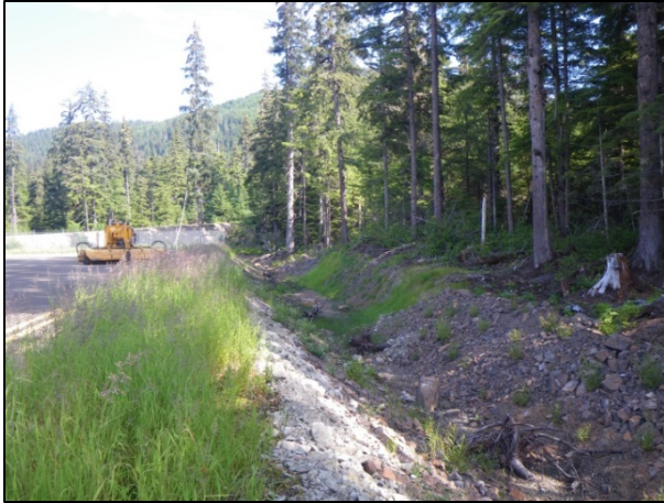
Figure 30.—Dry relocated reach, July 2014.
