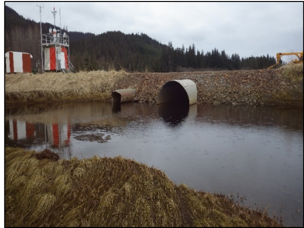
Figure 3.—Coho Creek culvert after installation, April 2015.
