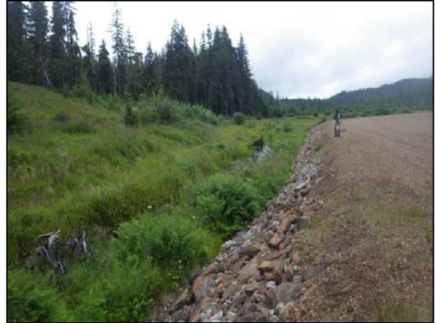
Figure 11.—Relocated reach, July 2017.
