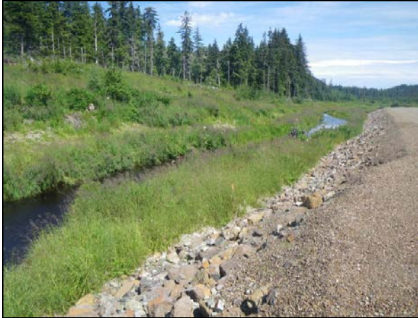
Figure 10.—Relocated reach, July 2014.
