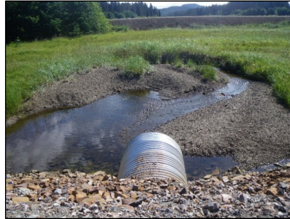
Figure 17.—Inlet of Shotter Creek culvert post-construction, July 2014.
