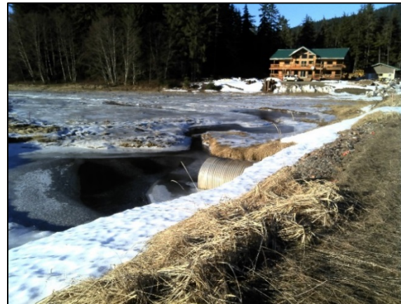
Figure 19.—Outlet of Shotter Creek culvert post-construction, February 2014.
