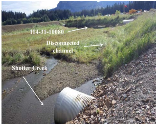
Figure 1.—Mainstem of Shotter Creek channel disconnected from Stream No. 114-31-10080.
