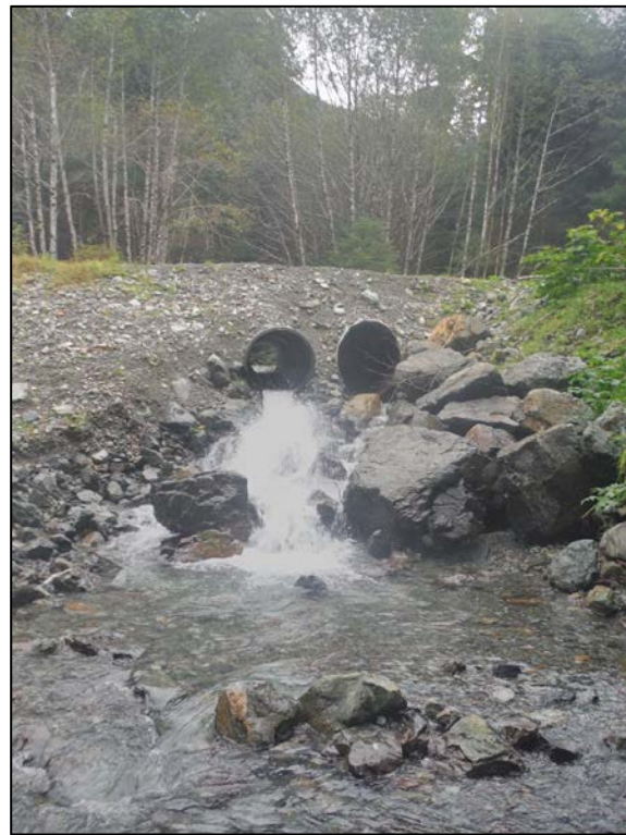
Figure 2.–Upper extent of Stream No. 113-41-10260 and Green Lake Road crossing.
