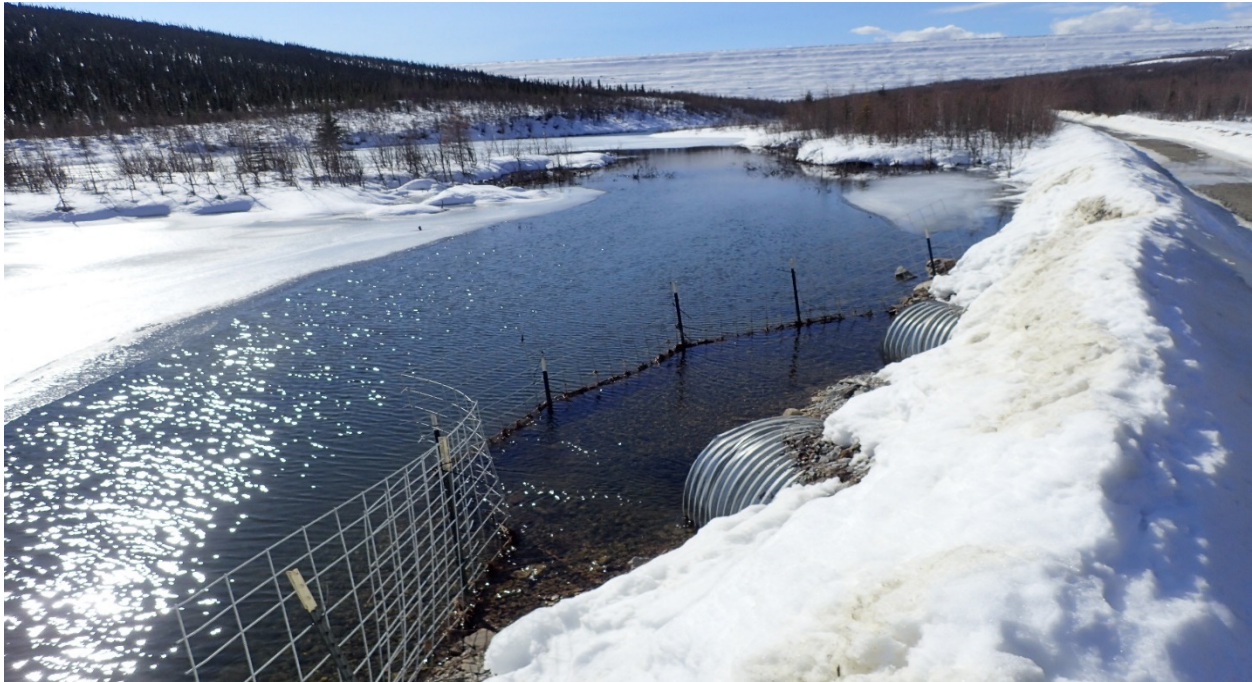
Figure 4. Beaver diversion fence installed at Pond AB culverts, April 15, 2021.
