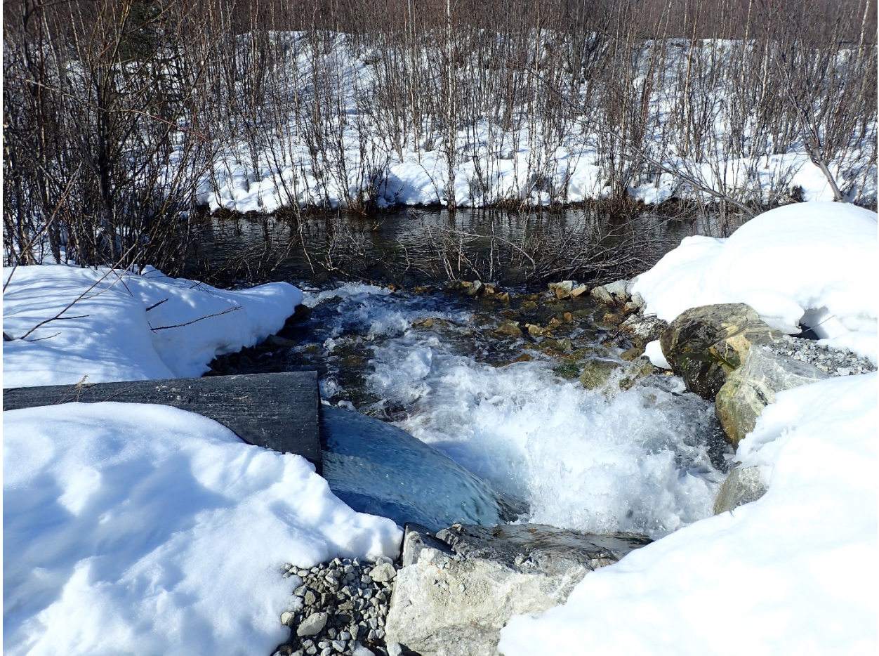
Figure 3. Outfall 002 showing RO water discharge of up to 3,000 gpm into North Fork Fish Creek, April 15, 2021.
