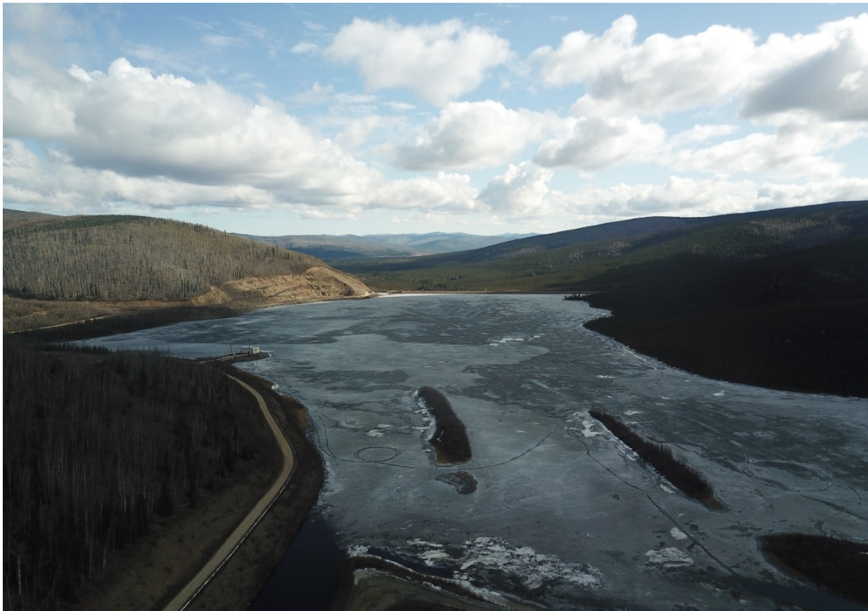
Figure 2. Fort Knox Water Supply Reservoir (WSR) May 2021.
