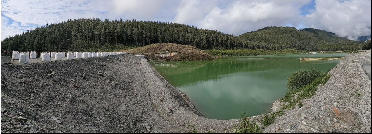
Figure 3.—Tailings Treatment Facility and Dam, August 26, 2021.
