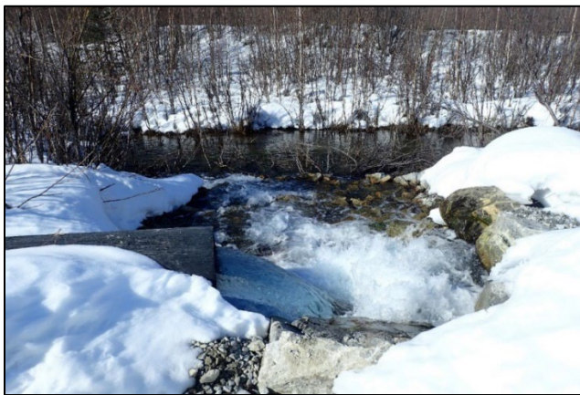
Figure 4. Outfall 002, RO water discharge of up to 3,000 gpm into the RO Channel Wetlands.
