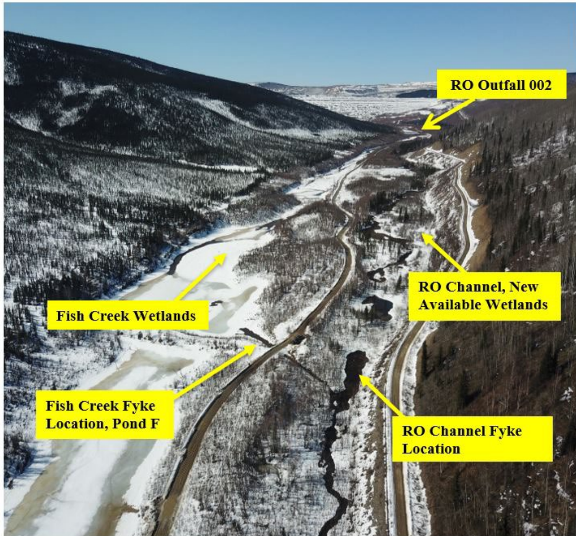
Figure 3. Fish Creek Wetlands Left, RO Channel Wetlands Right.
