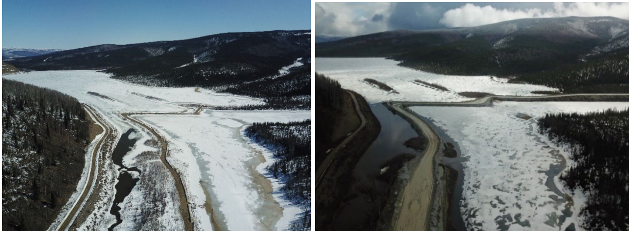
Figure 2. Fort Knox Water Supply Reservoir (WSR) and Gil Causeway, May 2020 (left) and May 2022 (right).
