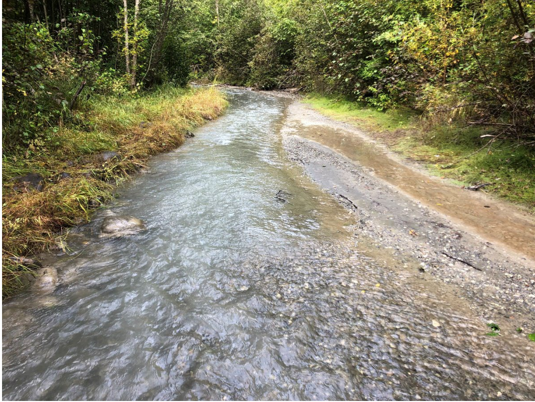
Eklutna 8 looking downstream – August 31, 2021
