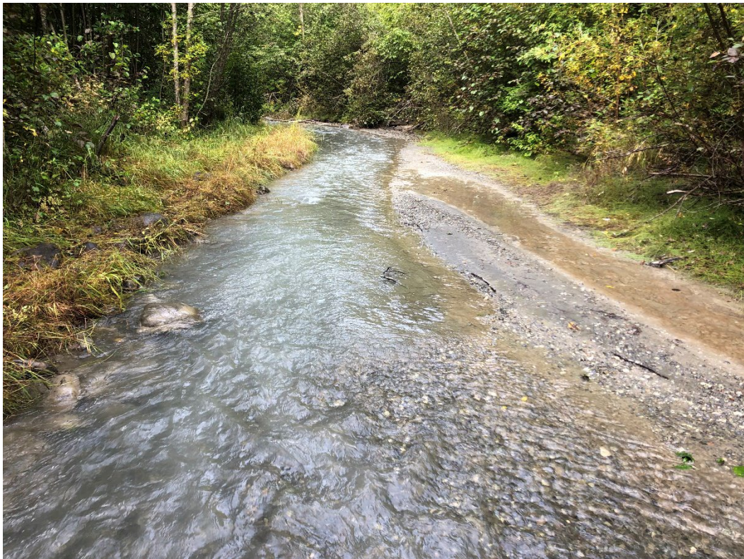
Eklutna 8 looking downstream – August 31, 2021
