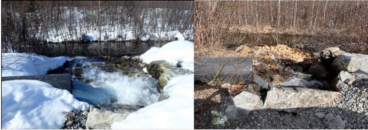
Figure 4. Outfall 002, RO water discharge of up to 3,000 gpm (2019 – 2021 left) and reduced to 800 gpm (2022 – 2023 right) into the RO Channel wetlands.
