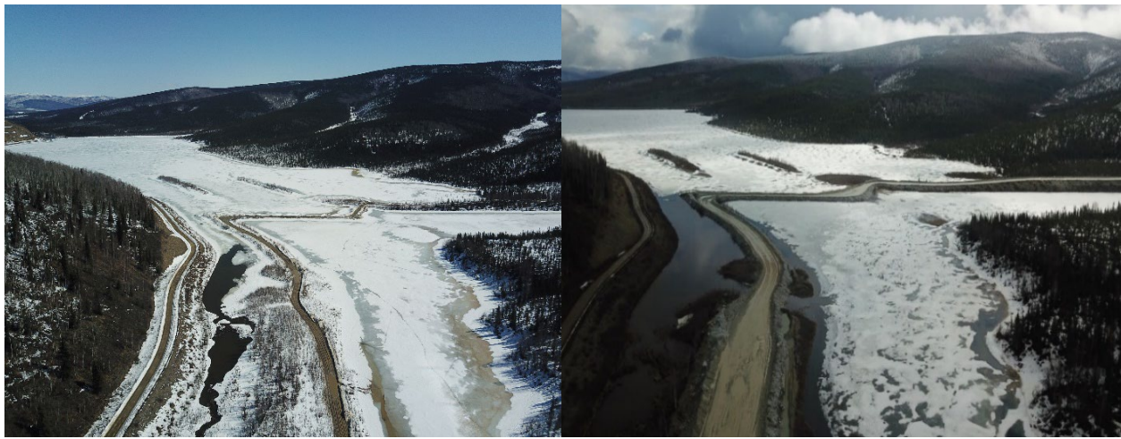
Figure 2. Fort Knox Water Supply Reservoir (WSR) and Gil Causeway, May 2020 (left) and May 2022 (right).
