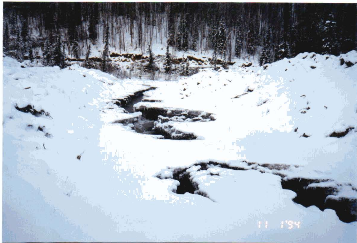
Figure 13. The freshwater diversion channel ice damming and overflow (top photo) and after flows had cut a new channel covered with fresh ice and snow (bottom photo).
