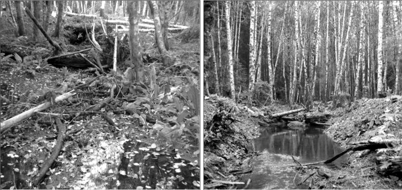
Figure 2.2. Before and after pictures of a blast site. Photos taken from the same perspective. Left photo shows a failing log culvert. Right photo shows the same location 2 years later.
