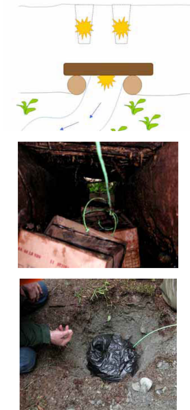
Figure A1.4 Box log culvert explosive design. Top: explosive placement for removing a box log culvert. Middle: boxes of emulsion are placed beneath the structure and connected to a detonating cord loop. Bottom: ANFO is buried deeply in the road fill and tied into detonating cord
